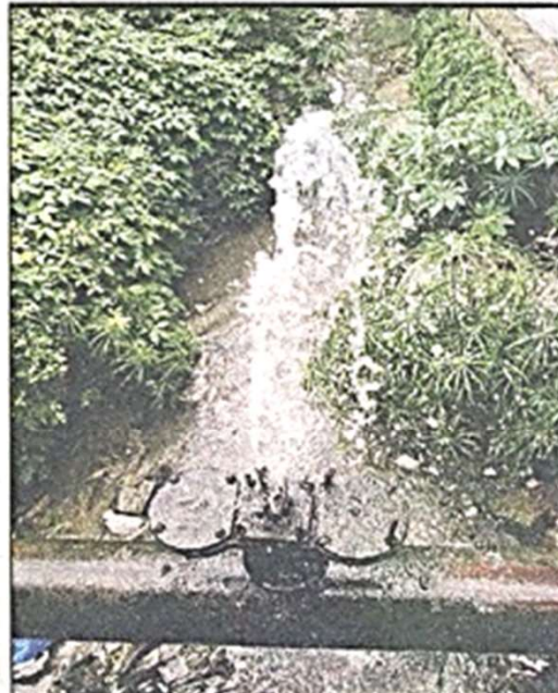
NOT UP TO MARK: BWSSB loses 44% of water to pilferage and leakages
