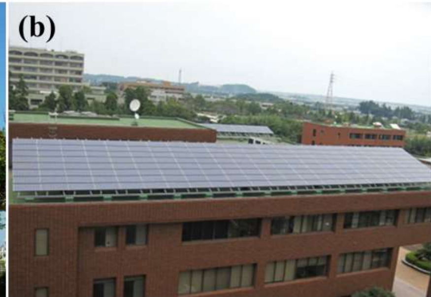
(a) Wall-mounted Si PV system and (b) 20° tilted Si PV system. Both systems were installed facing south at the University of Miyazaki.
