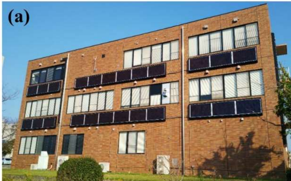
(a) Wall-mounted Si PV system and (b) 20° tilted Si PV system. Both systems were installed facing south at the University of Miyazaki.
